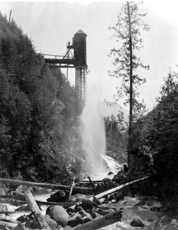
Figure 3. Coffee Creek Showing Water System
