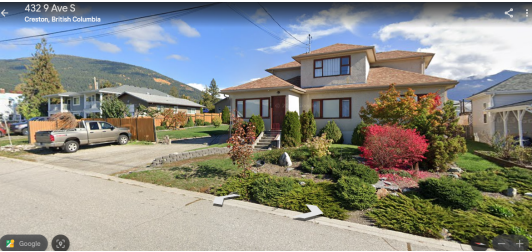
Figure 1. House built by my father L.S.R. /n a
